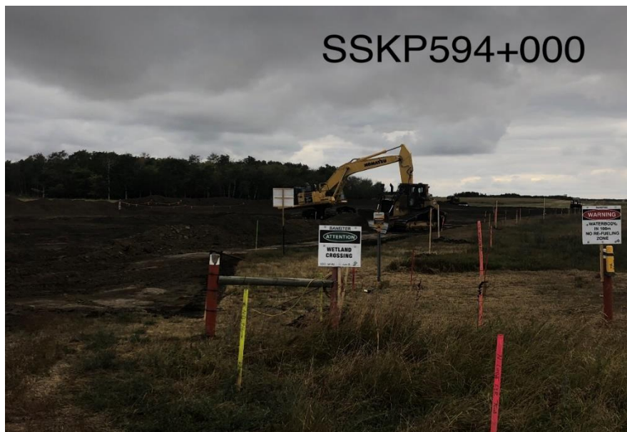
Top soil stripping near wet land crossing
