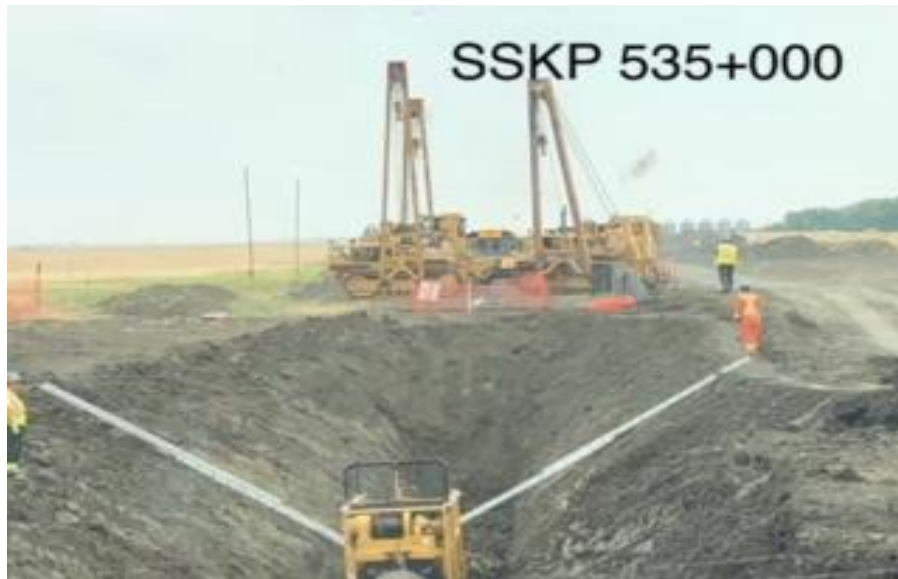
Bore through road by track bore
