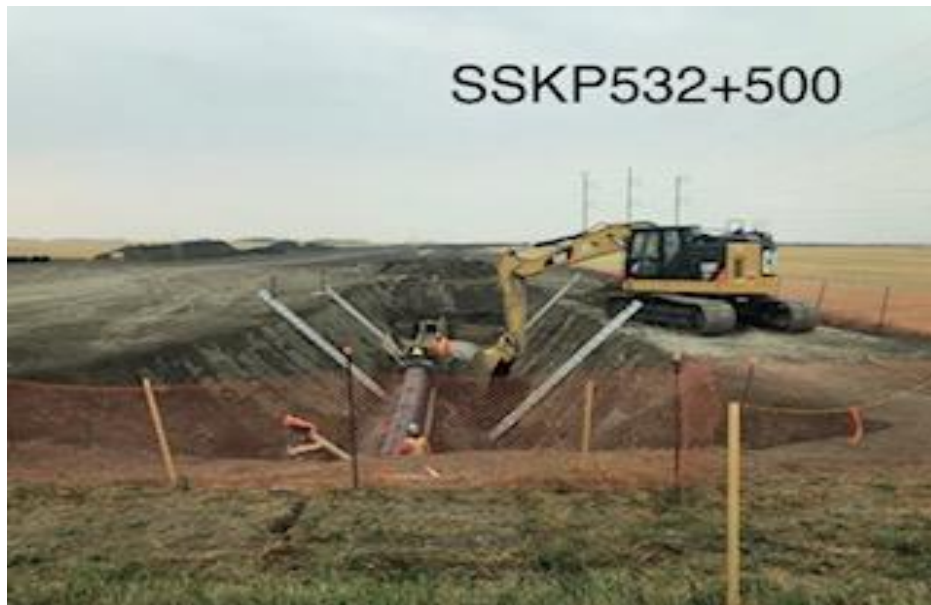
Track bore installation at shoofly 2
