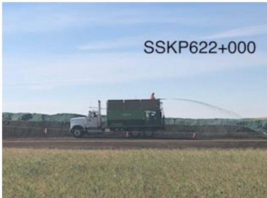
Crews continue to apply ditch spoil separation layer
