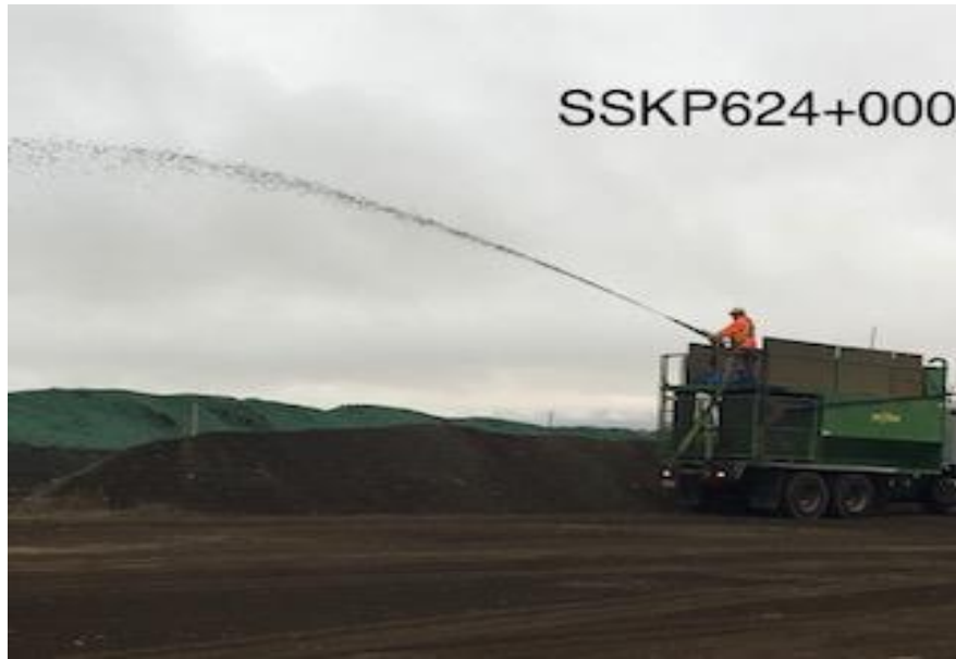
Ditch soil separation layer being applied at Chapleau Lake
